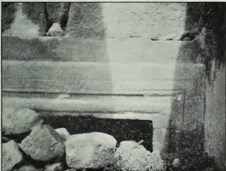
FIG. 104.—No. 16, door between narthex and nave, from W.
